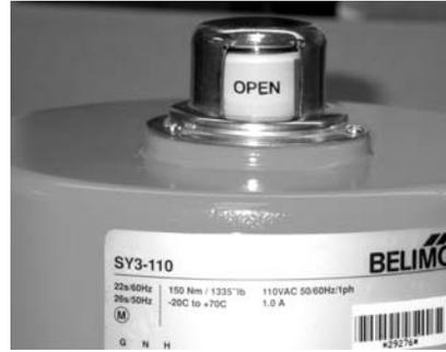
**Step 7)** The SY actuator is shipped in the OPEN position. Make sure the actuator is in the OPEN position before attaching to the valve/coupling assembly. The SY actuator turns counter clockwise (CCW) to the OPEN position, when viewed from ABOVE the actuator.
