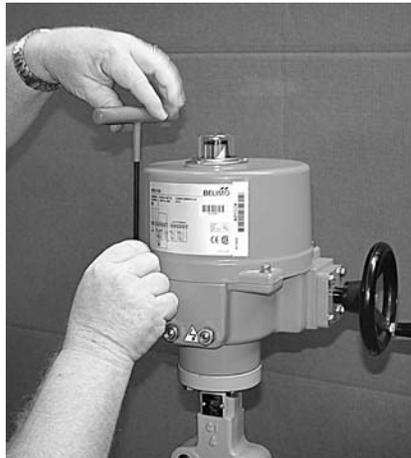
**Step 1)** Remove the four hex bolts securing the cover to the base casting.
