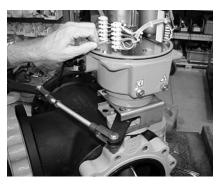
Step 25) Using the correct control signal (On/Off or Proportional) drive the MASTER valve 25% CLOSED, then drive the MASTER valve fully OPEN. The SLAVE valve should now be fully CLOSED. The SLAVE valve should now be fully CLOSED. If the
