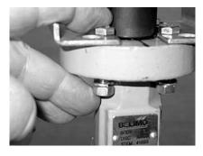
**Step 6)** Insert the four mounting bolts (B), lockwashers (C), and the hex nuts (D). Do NOT tighten at this time.
