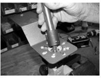
Step 3) Determine the position of the valve disc. Most manufacturers mark the TOP of the valve stem with a slot which indicates the disc angle. Slide the drive pin assembly, consisting of the drive shaft (E), the valve
