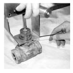
STEP 13) Once the linkage is fully seated on the valve bonnet, tighten three setscrews (G) in the collar to affix the linkage onto the valve.
