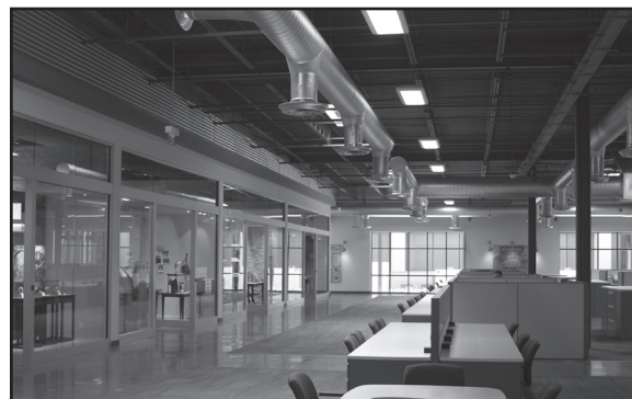
TMR diffusers installed in an open ceiling office environment
