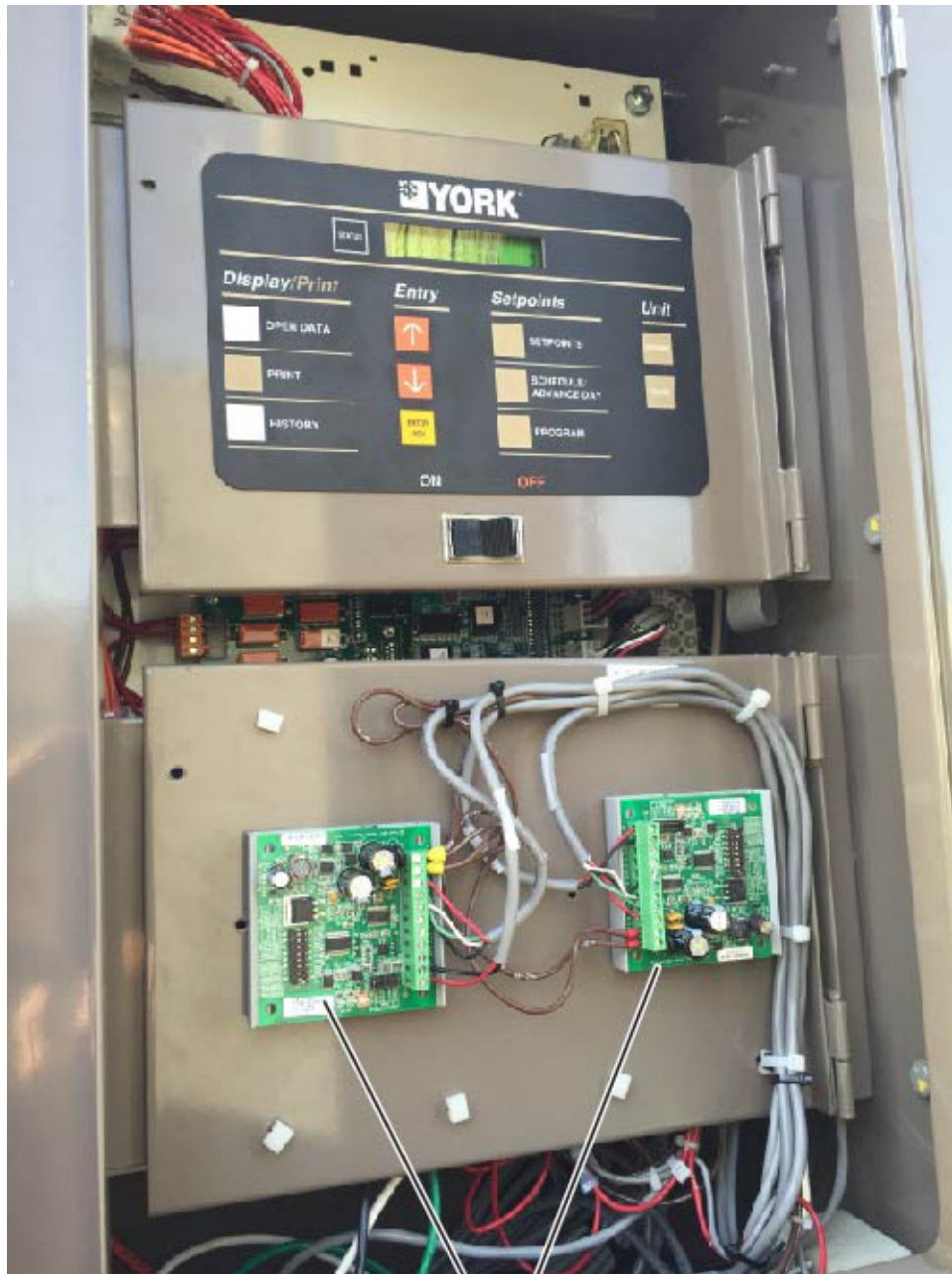
MOUNTING LOCATION OF THE SPORLAN (PARKER) CONTROLLERS
